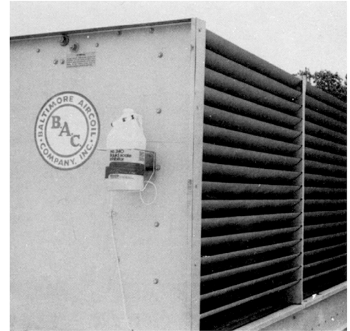
Arrange Drip Feeder so that lower end is about 1 inch below surface of sump water.
